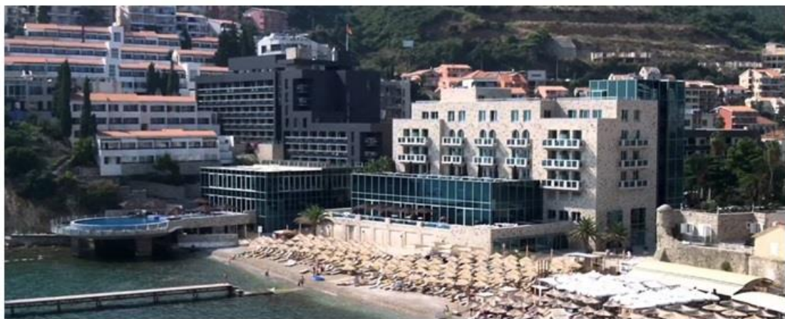
Figure 4.4: Reconstructed Avala. The number of hotel’s buildings increased (see the left side), the number of floors and change its visual identity. The main part is now larger than Old Town Walls (see the right side). (Asmec Consultants, n.d)
