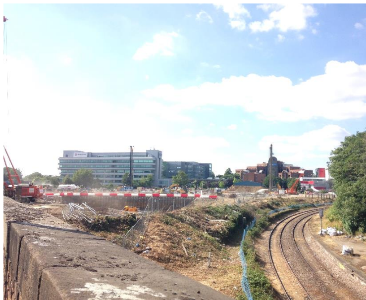
Figure 2: The construction site at Lionel Road
