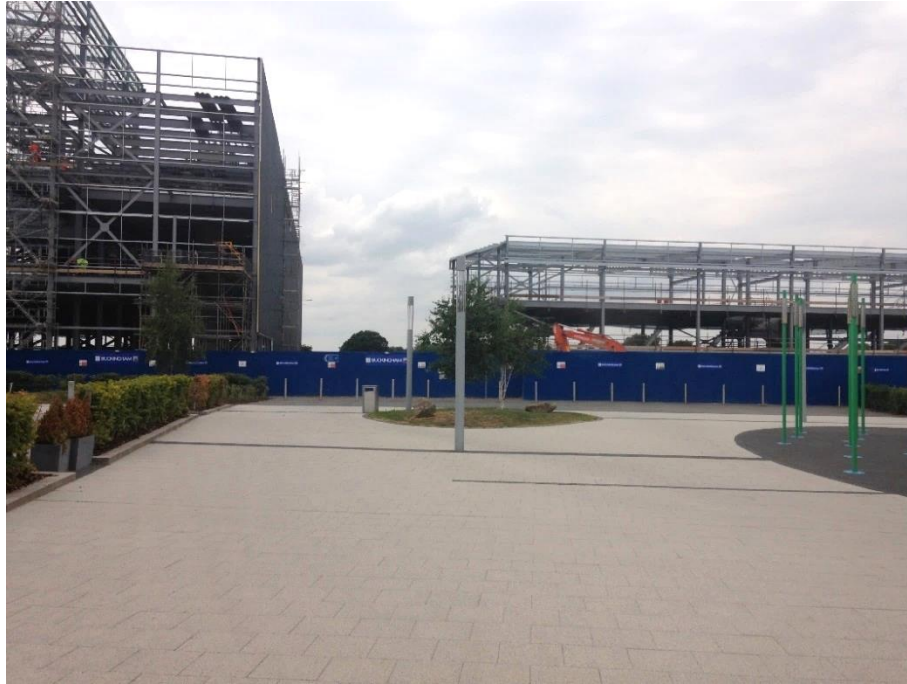
Figure 12: York Community Stadium’s gateway entrance under construction. Source: Author (2018).
