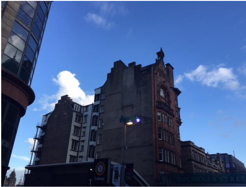
Figure 21: Wall in Buchanan Street.
