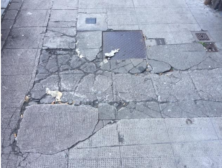
Figure 8: Cracked pavement.
