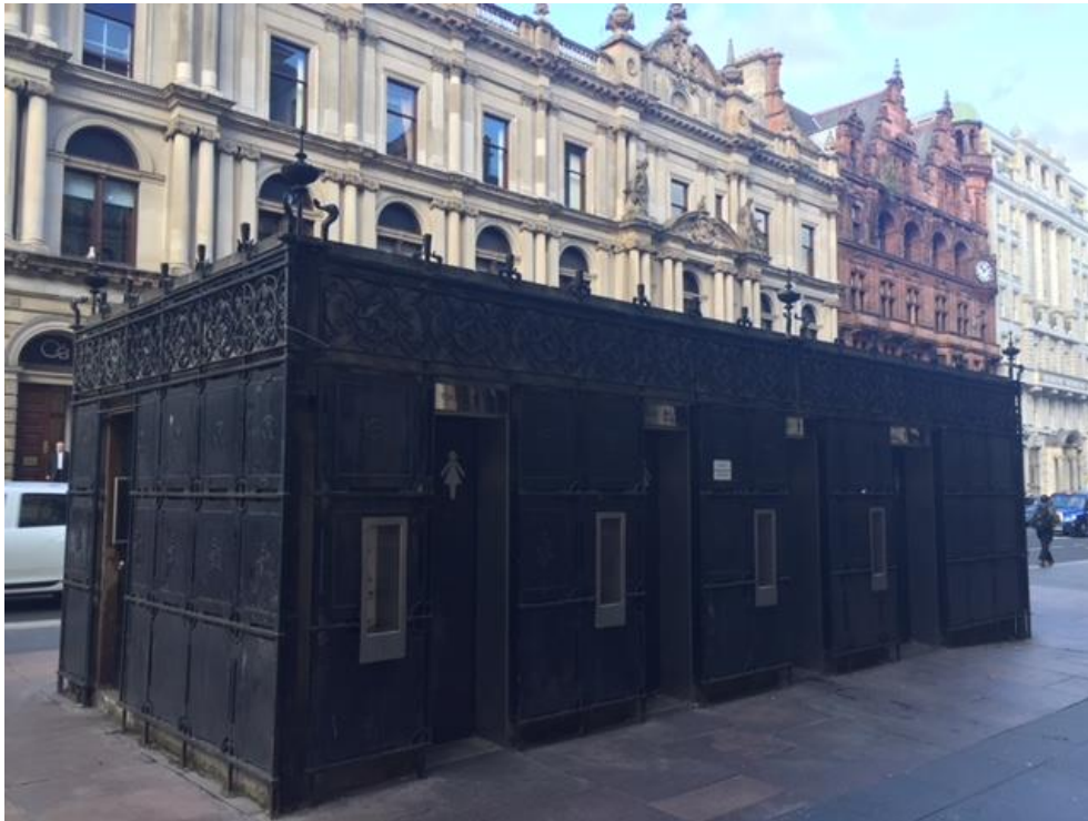
Figure 28: Public Toilet on Buchanan Street.
