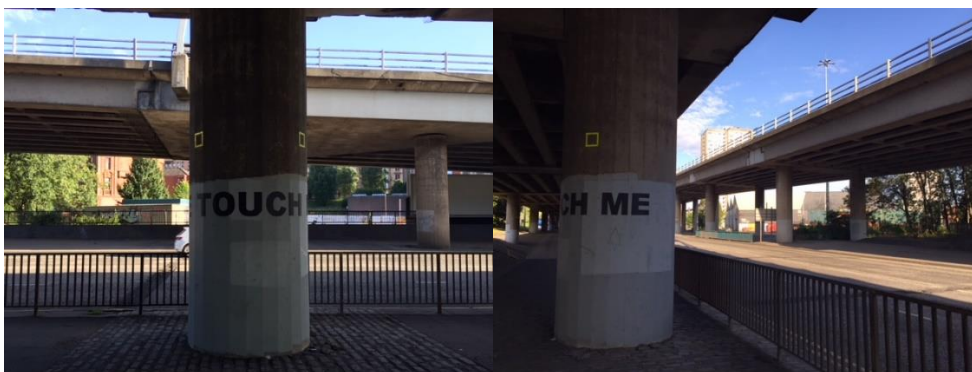
Figure 34: Pillar below the M8 motorway reading: 'Touch me'.
