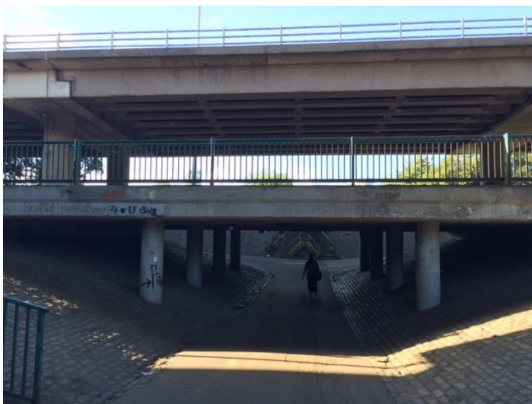
Figure 35-37: Walking through the underpass.
