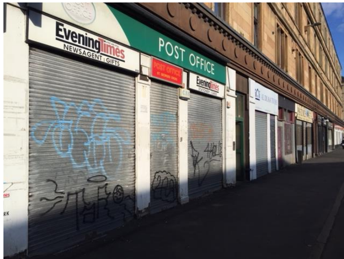
Figure 20: Graffiti-tagged, run down garage door.
