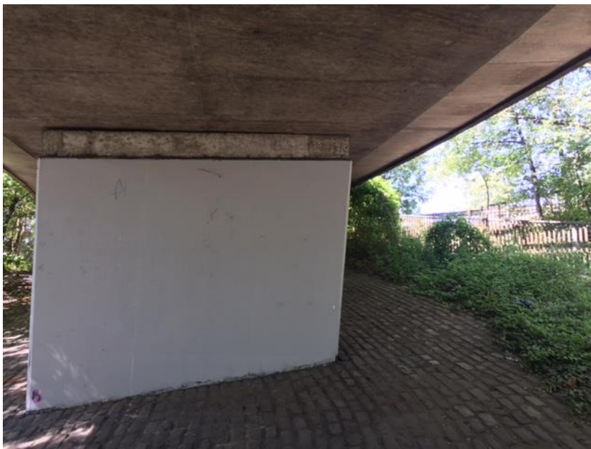
Figure 22: White wall under the M8 bridge.
