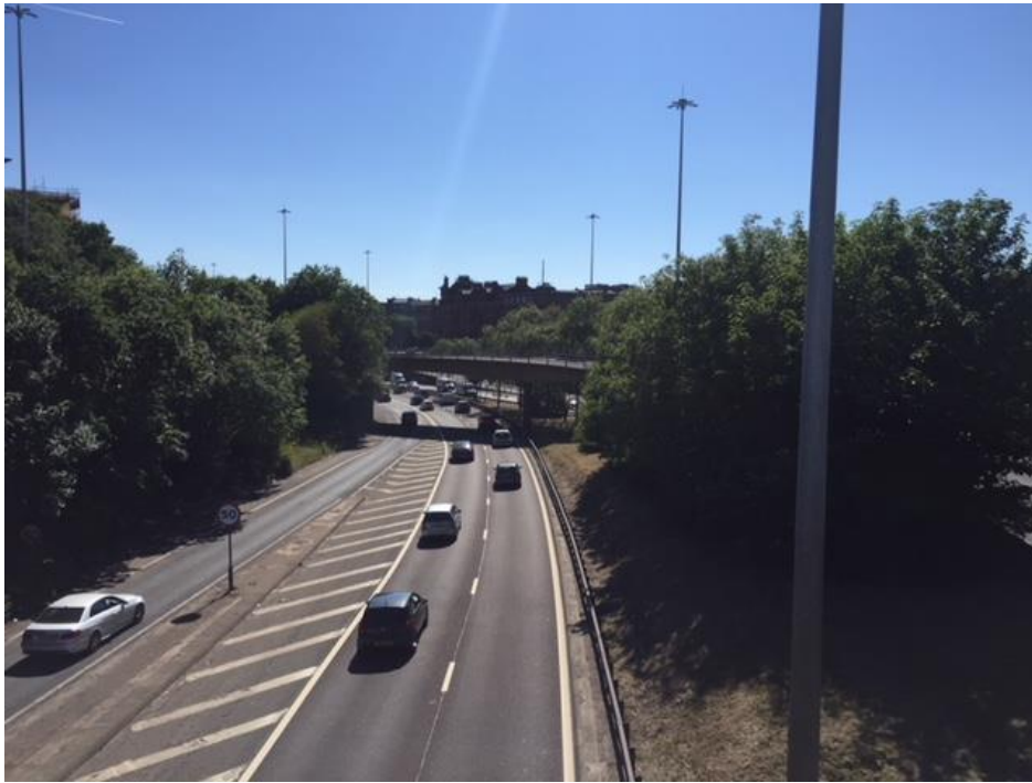
Figure 42: Looking down from the walkway over the motorway.
