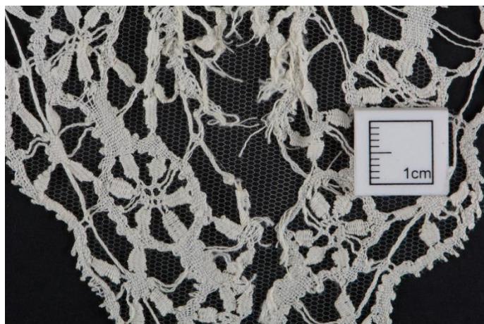
Fig. 8.4.2 Area of damage A after supporting with a 20-denier nylon net patch.
